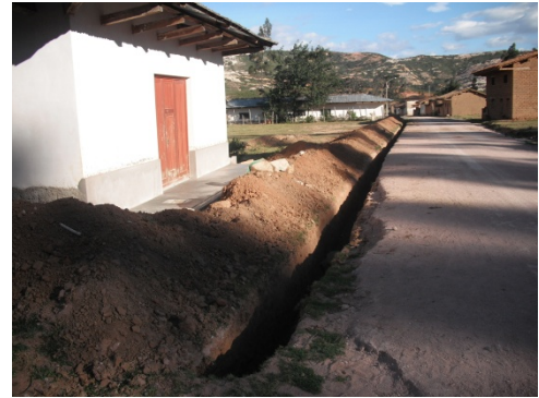
Installation of electricity and water in the Sexi museum building
