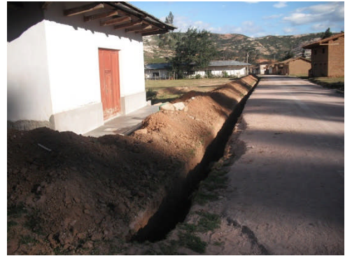
Installation of electricity and water in the Sexi museum
