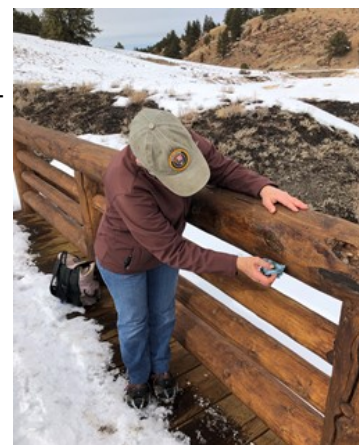
Volunteer Mary Capps repairing splintered handrail on the footbridge near the Homestead
